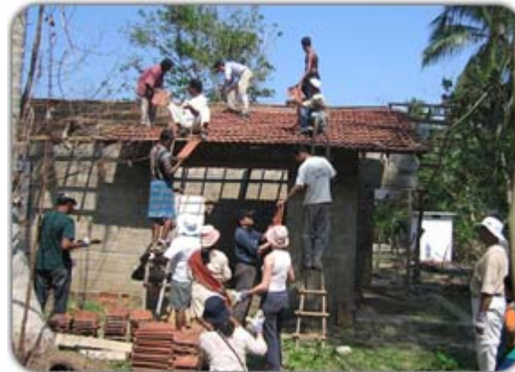
Staff hard at work on the Wilbert Mendez house.
